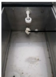
Water shortage level sensor
