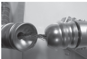
Figure 8 – Cable demonstrating fatigue and fraying
